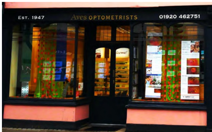
Figure 36- Appropriately scaled lettering to height of fascia.
