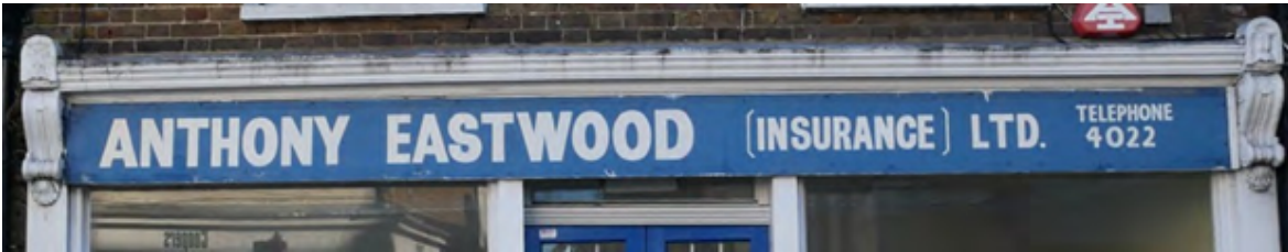
b) The sign has been located within the fascia area, contained by the corbel. It would have been more successful if painted onto the wooden fascia boards with the main name reduced in size.
