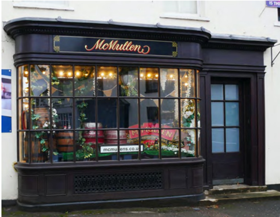
Figure 28 - A well-balanced frontage with stallriser of an appropriate height.
