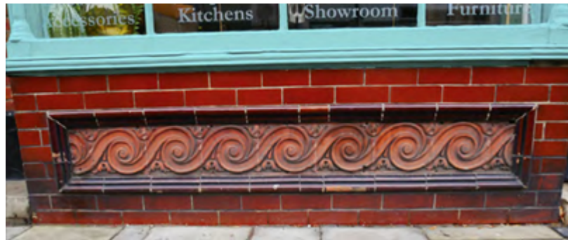
Figure 29 - Tiles with moulding and terracotta to the stallriser.
