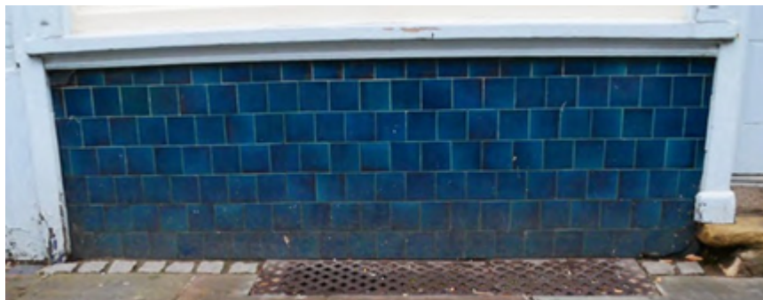
Figure 30 - Glazed blue tiles appropriate to this stallriser.
