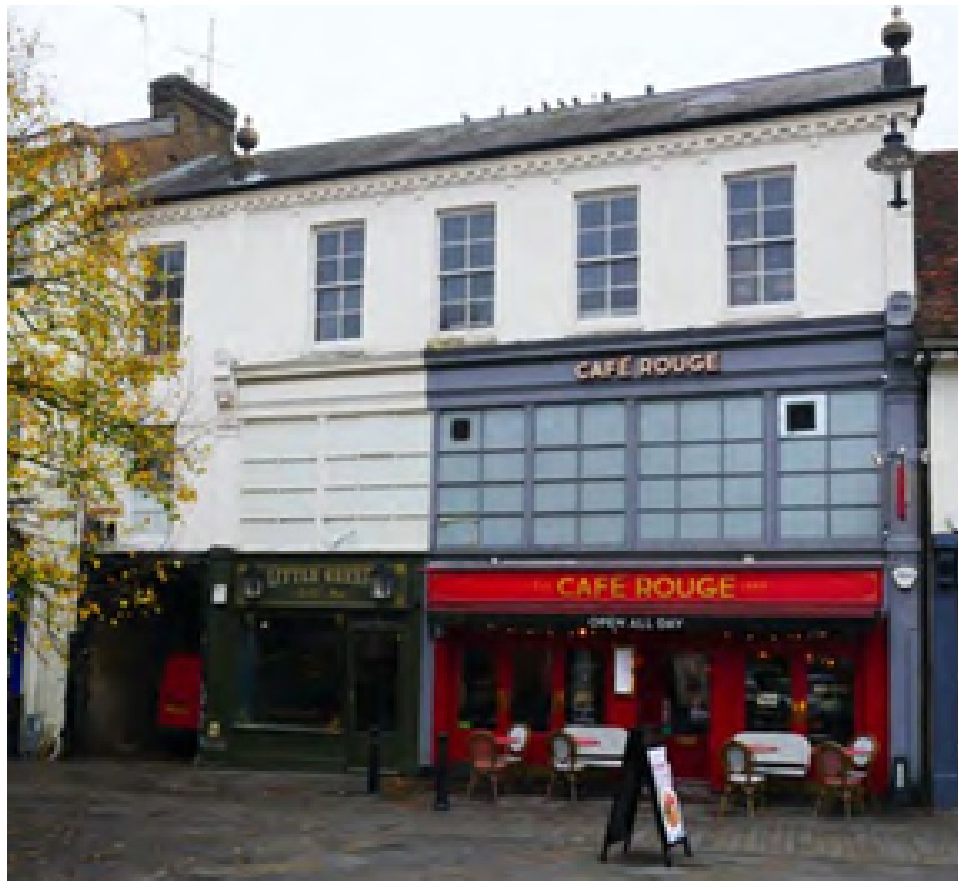
Figure 18 - late 19th century Emporium with multi-paned display windows to first floor with altered 20th century timber shopfronts.
