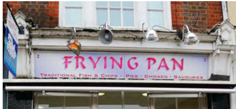
Figure 40 – Unnecessarily extensive lighting.
