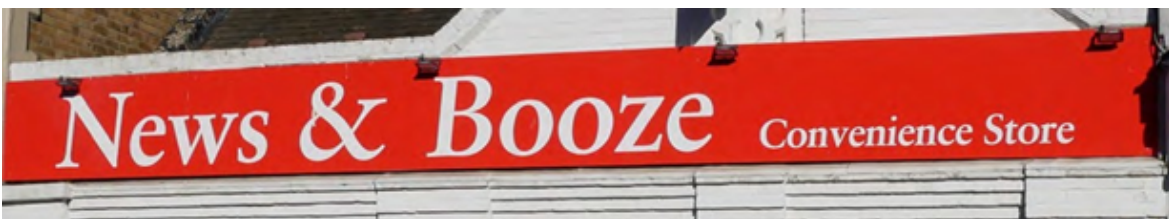
d) A plastic fascia board that is overly bright with large lettering and external lights that overpowers this building.
