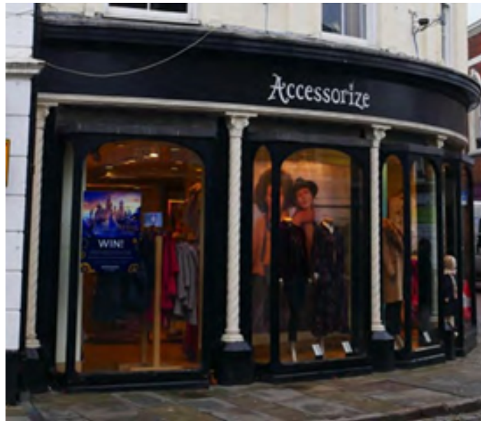
Figure 21 – The identity of a chain store respecting the style of the curved shop with its fascia supported on barley twist columns with plinth and ornate capital.
